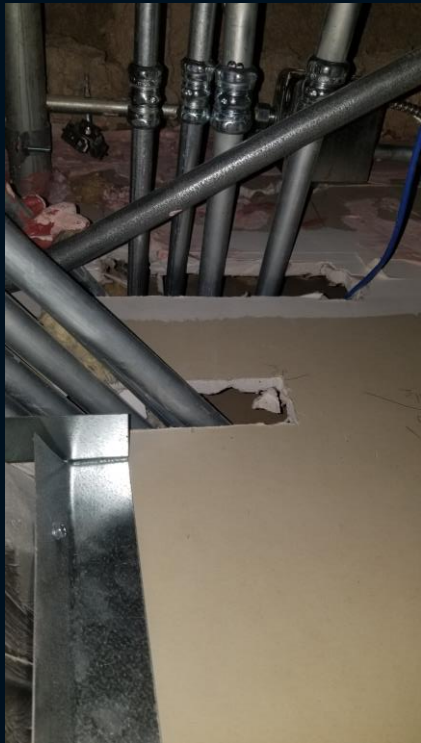
No Wall Labels & No Fire Stopping
