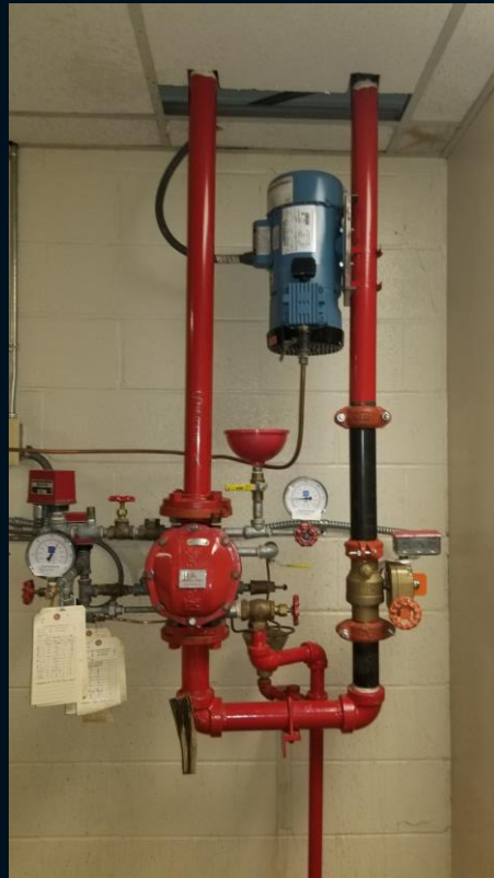
No Valve Labels To Indicate Area Served
