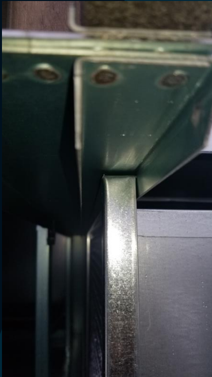
No Gaskets Final Filters
